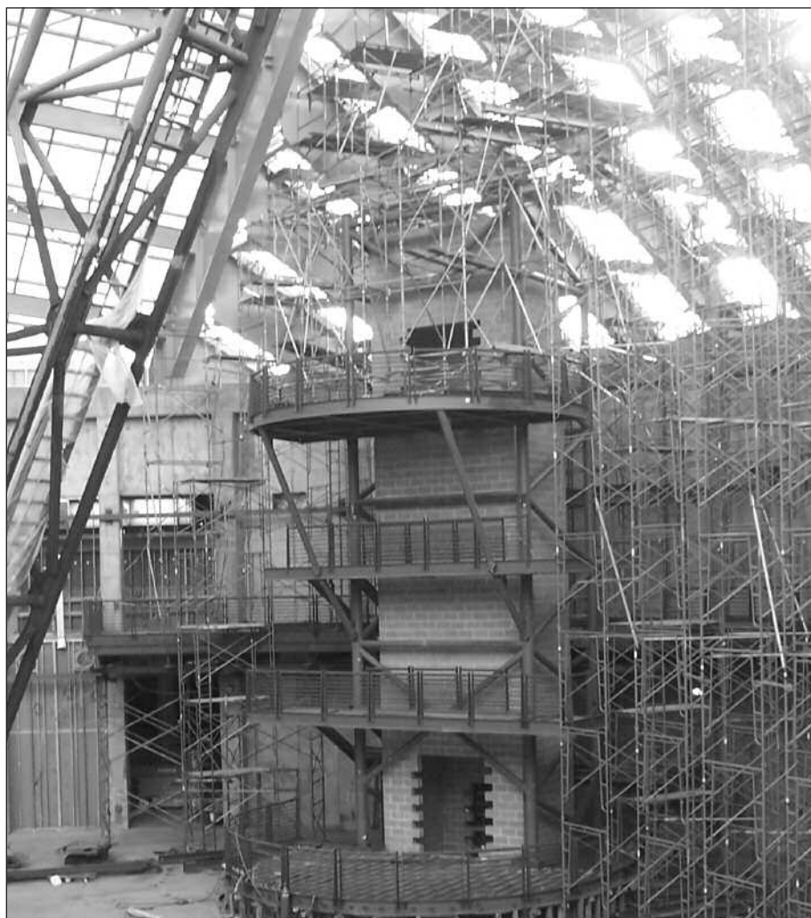
Interior detail of the National Museum's Central Gallery shows viewing platforms that evoke the bridge decks of an amphibious assault ship.
